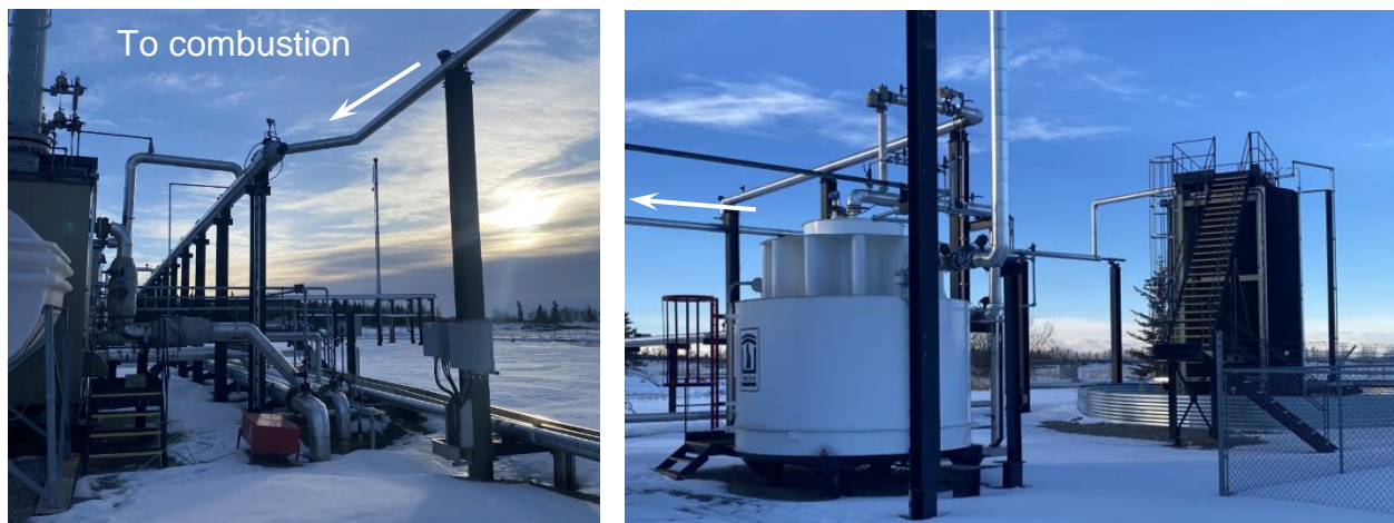
Figure 17: Condensate and water tank with vapour recovery tied into flare and combustor
