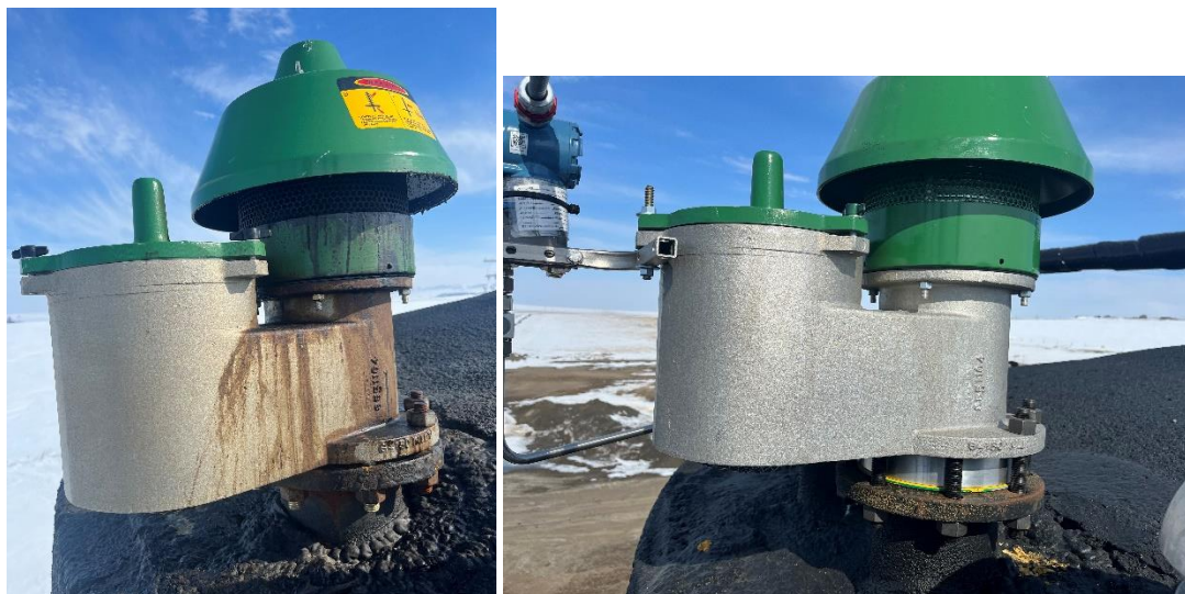
Figure 3: PVRV with pressure sensing ring and wired pressure transmitter added
