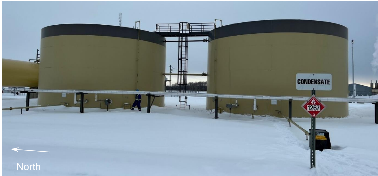
Figure 12: Monitored condensate tanks
