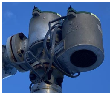
Figure 16: Site layout, thief hatches and pressure vacuum relief valves
