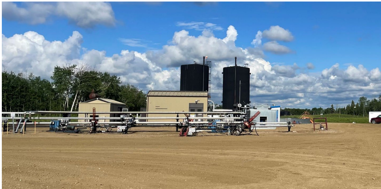
Figure 1: Typical Heavy Oil Multi-well Pad Site
