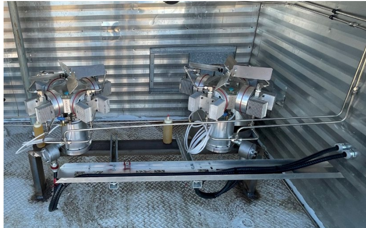
Figure 5: Installation of Prototype LCO VRUs
