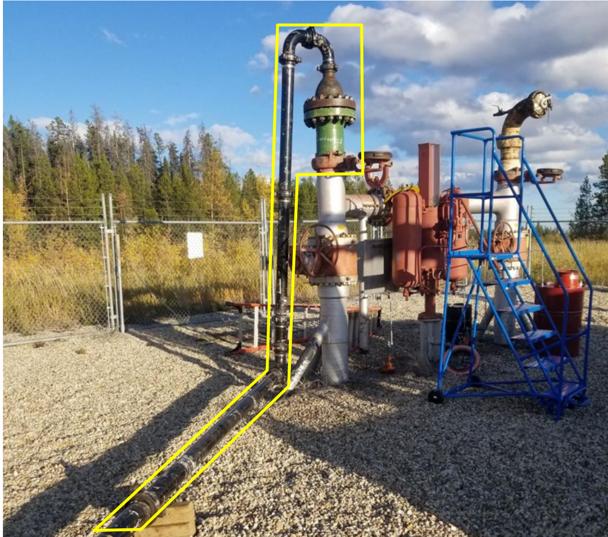
Figure 8: Tie-in point for Pilot #1.
