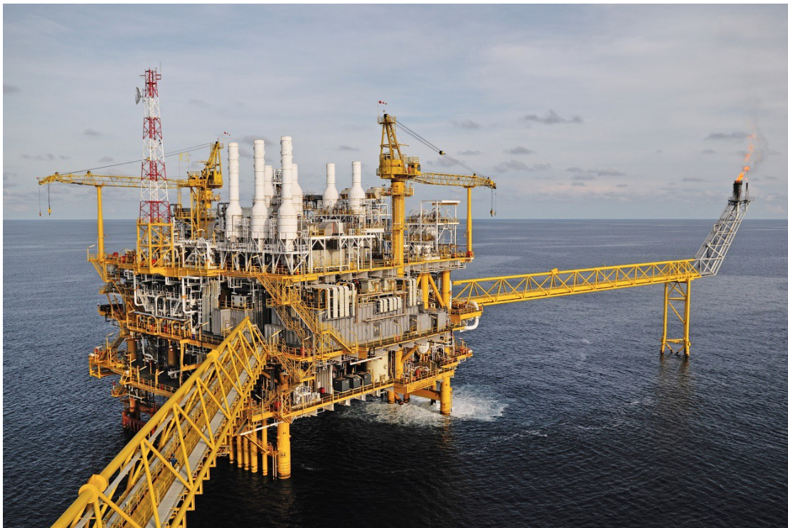
Figure 1.1 Typical offshore oil production facility
