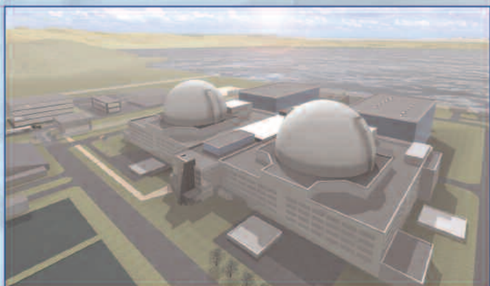
Artist's impression of a 2-unit ACR-1000 GEN III+ Nuclear Power Plant: 1200 MWe class
