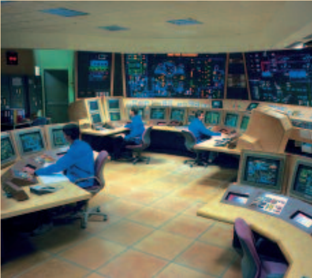
A computerized screen-based control room designed to maximize operator efficiency. Chooz B1, France (N4, 1,500 MWe).
