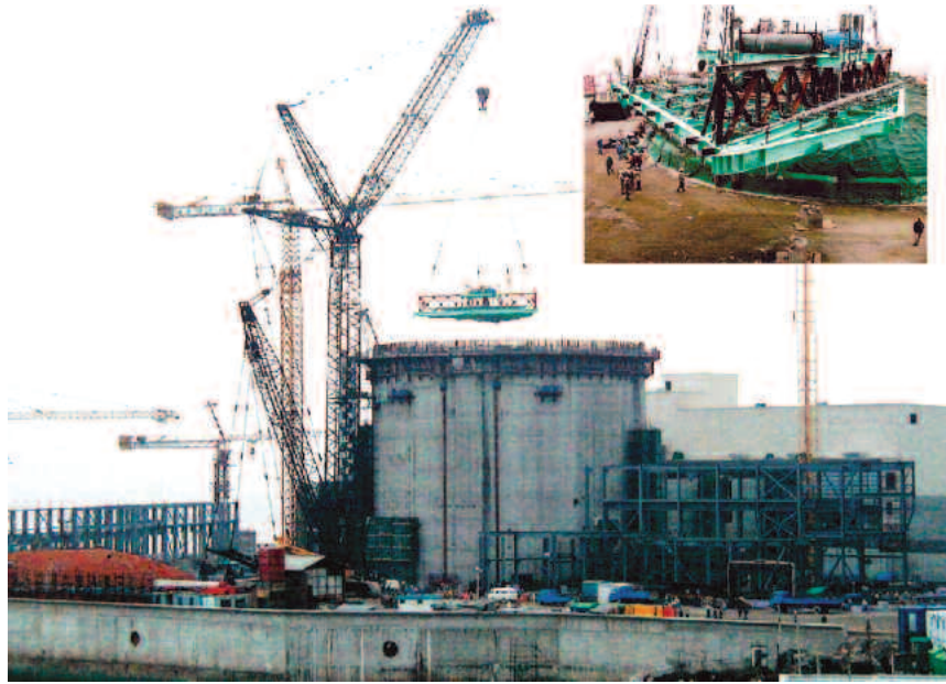
Figure 4-3 Module Lift Using VHL Crane
