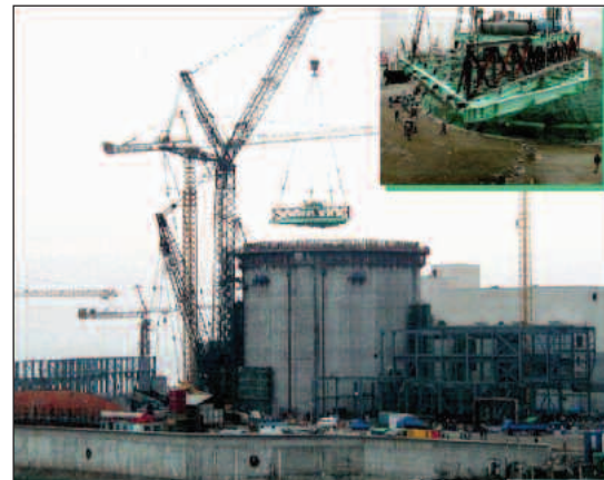
Figure 4-3 Module Lift Using VHL Crane
