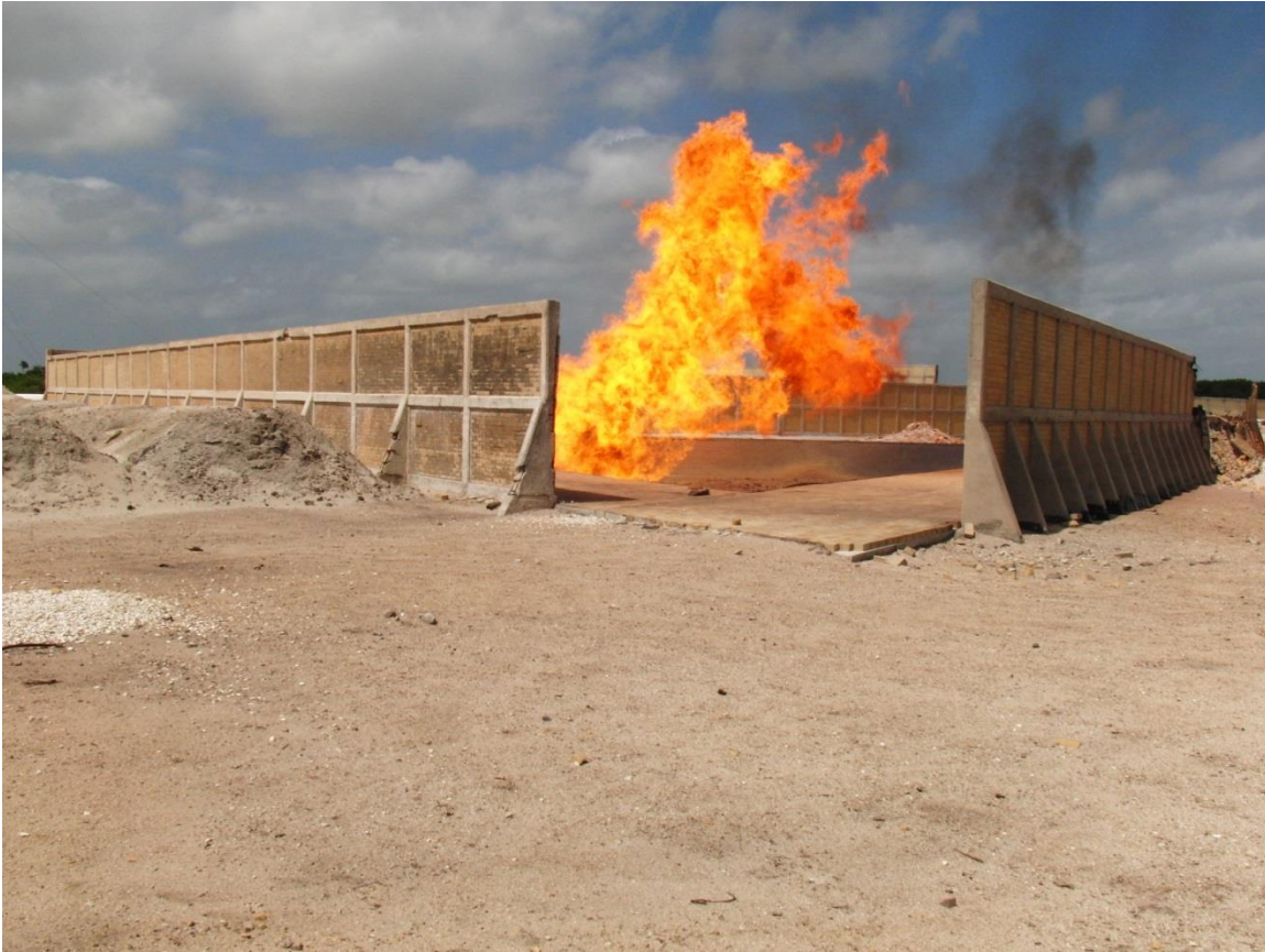
Figure A.1: Pit flare at the Atasta compressor station in Campeche, Mexico.
