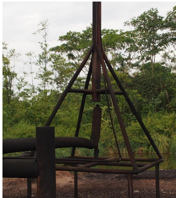
Figure B.14: Ambient air entrainment (premixing) technique using converging nozzle and vertically offset flare stack.
