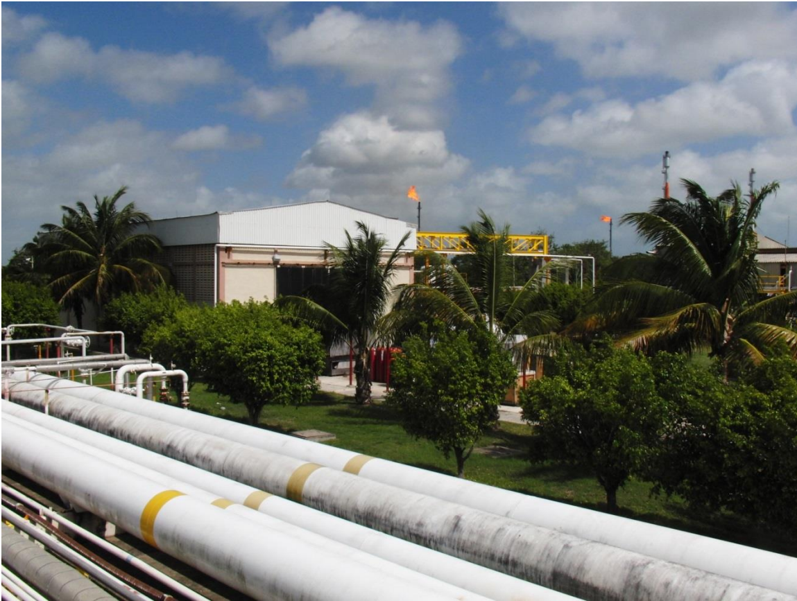
Figure A.3: Northern emergency flare (operational flare at the right of the image) at the Atasta compressor station in Campeche, Mexico.
