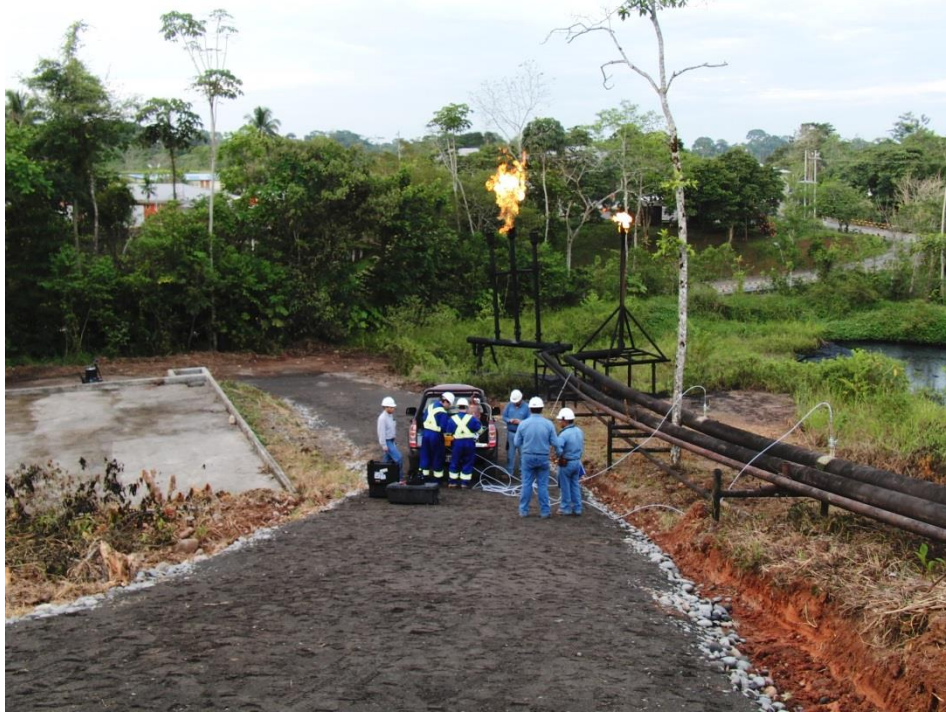
Figure C.8: Flares at Auca Central. Hot taps were available only for the line feeding the right flare in the image and only this flare was the subject of sky-LOSA BC and flow rate measurements.
