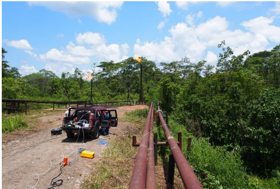
Figure C.4: Flares at Auca Sur. Both flares visible were measured as Auca Sur Right (pictured right) and Left (pictured left). The rightmost two lines had hot taps installed and fed the rightmost flare. Site staff informed Carleton personnel that the adjacent line was inactive, there were also no hot taps which precluded confirmation by measurement. The leftmost flare was fed by a single line which enters the lefthand side of the image.
