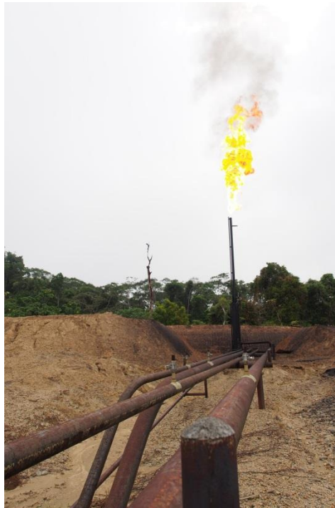
Figure C.2: The flare at Auca 27 had the largest flare gas flow rates of the measurement campaign. Pictured are the four lines feeding the flare, all of which were the subject of one or more flow rate measurements as well as extractive gas sampling.
