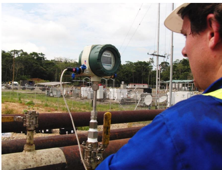
Figure B.8: Measuring flow with the constant temperature TFM at Auca 27.
