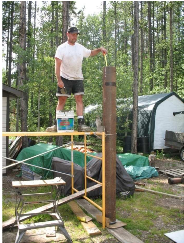
Checking Cement Plug Length
