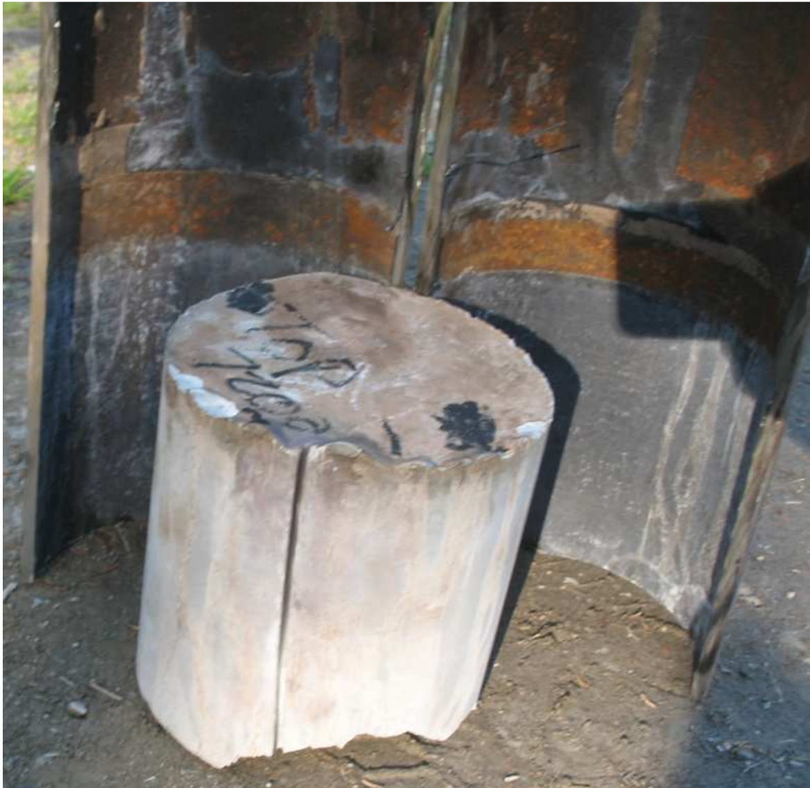
Sample 7200 Top Of Cement Plug And Pipe
