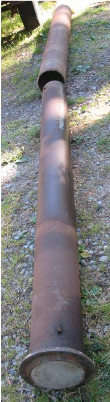
Sample 7200 Cut And Pulled Apart
