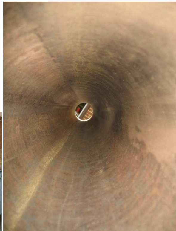
Cleaned Pipe Surface
