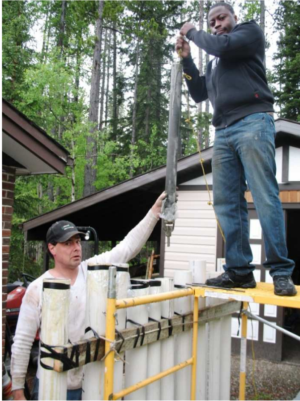
Compression Test Samples – Placing Cement With Dump Bailer
