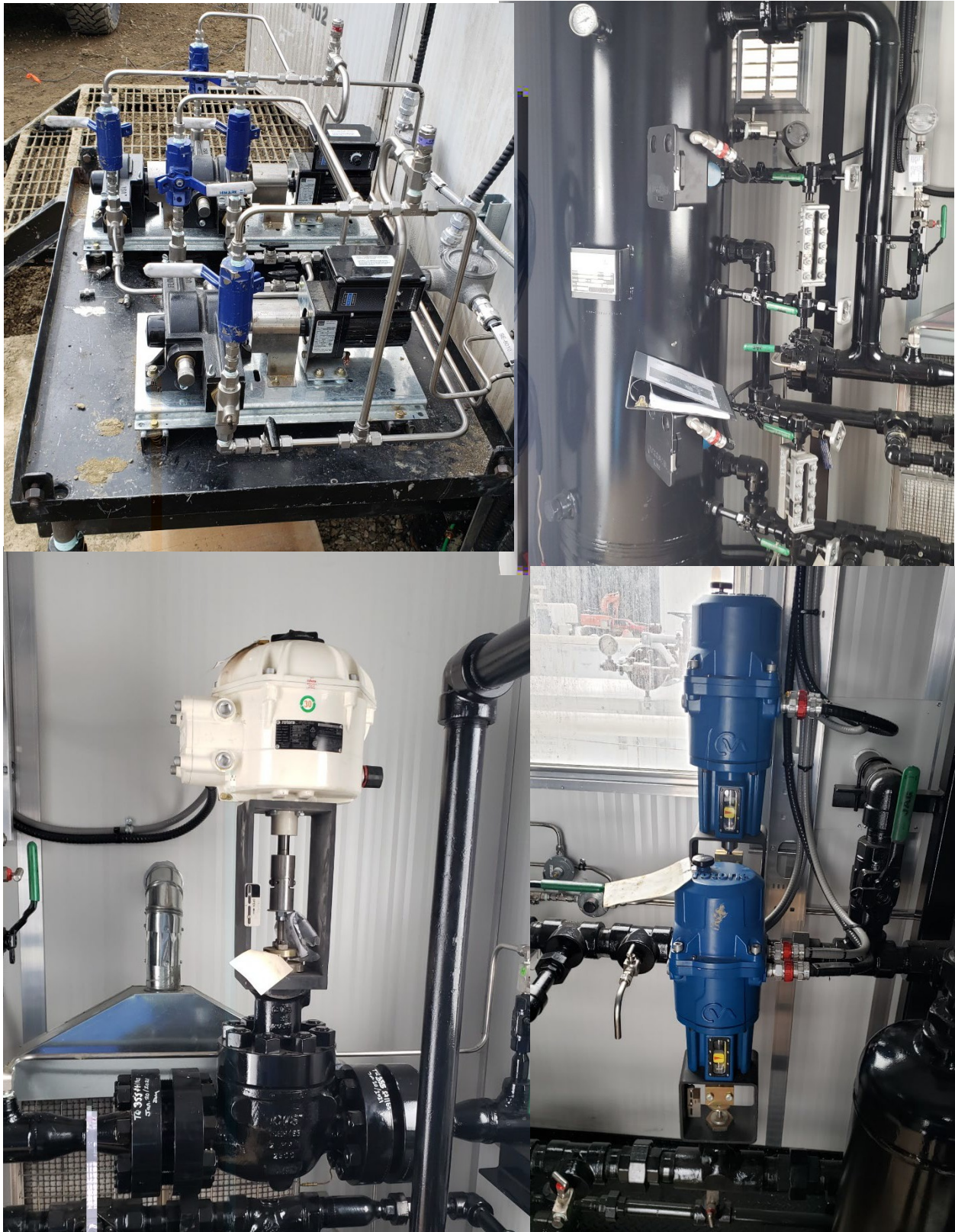
Figures 5-8: Electric Package B – [clockwise from top left] (5) Flomore Ecoflo 35 electrical chemical injection pumps, (6) Norriseal 1001A electric level controllers, (7) Rotork CML 750 FA05 level control valve actuators, (8) Rotork CVL1000 FA07 inlet control valve actuator
