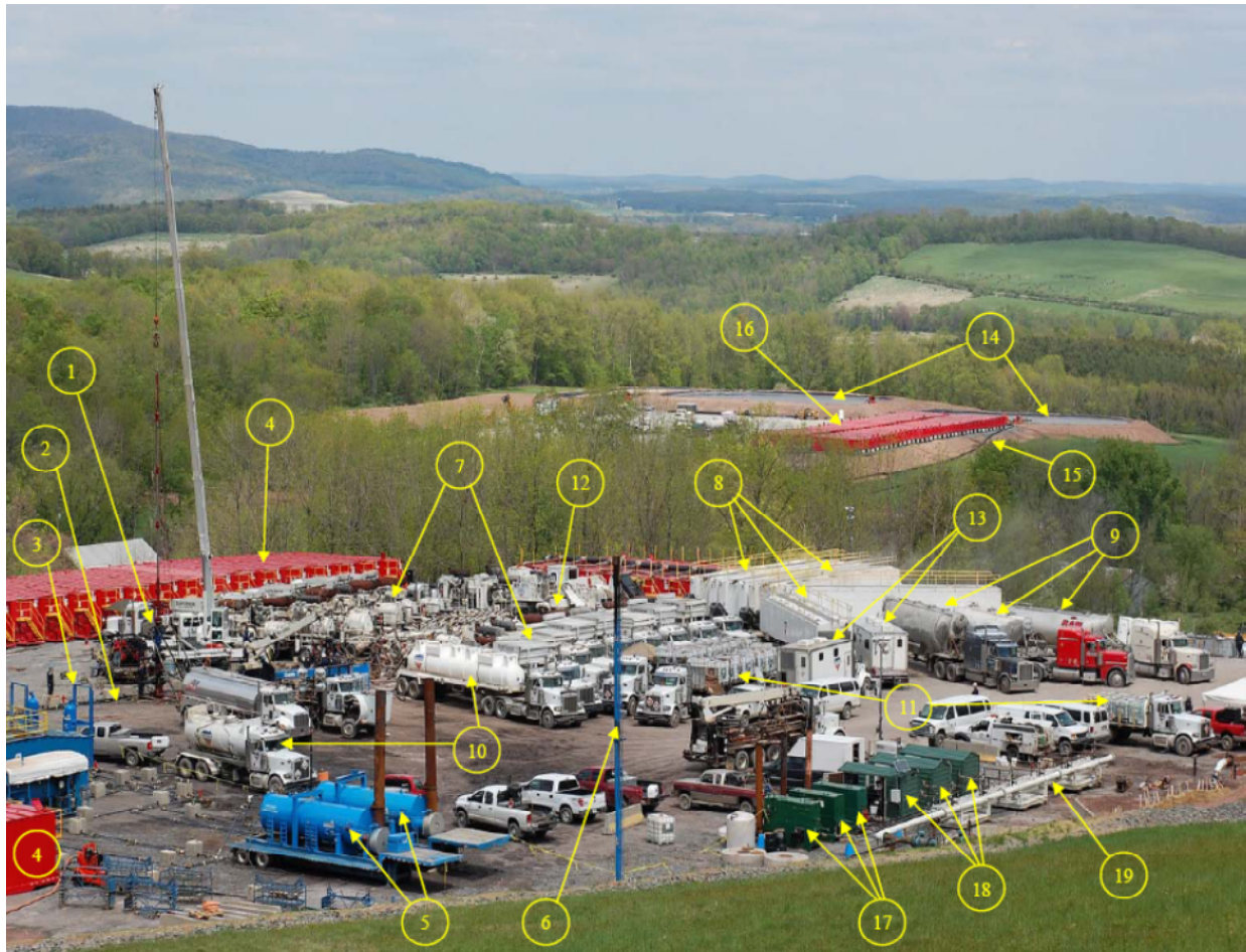
Figure 5 Equipment Setup For Hydraulic Fracturing (Source Doc 4)
