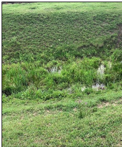
Figure 3-1: Standing water site conditions, MP 27.5276
