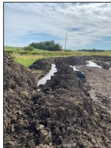
Figure 3-2: Standing water site conditions, MP 29.52
