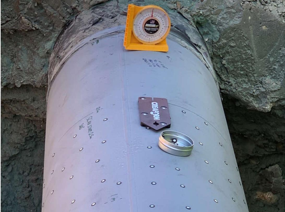
Figure R: Surface Preparation for Laser Scanning of Features
