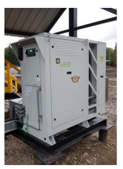
Further efficiencies can be realized by using waste heat (about 3 times the power rating) as a heat source for additional hot glycol.
