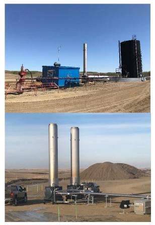
A small continuous pilot that uses less than 100 scf/d of fuel gas allows for stable combustion of intermittent flows as soon as the vapours enter the combustion chamber.
