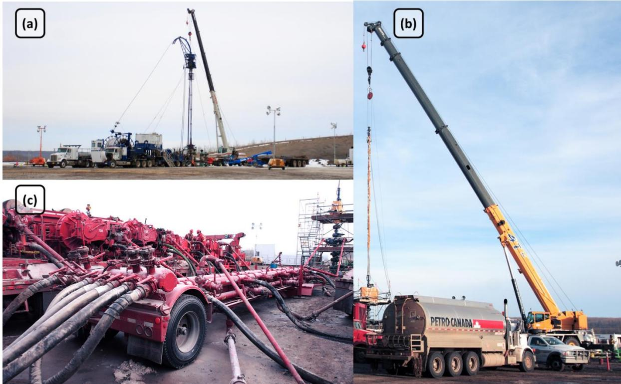
**Figure 4.6: (a) Coil tubing operation drilling out stage plugs, (b) Onsite fuel delivery, (c) Pump trucks for fracturing fluid**
