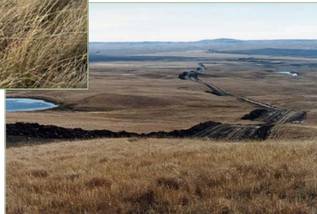
Pipeline through fescue grassland
