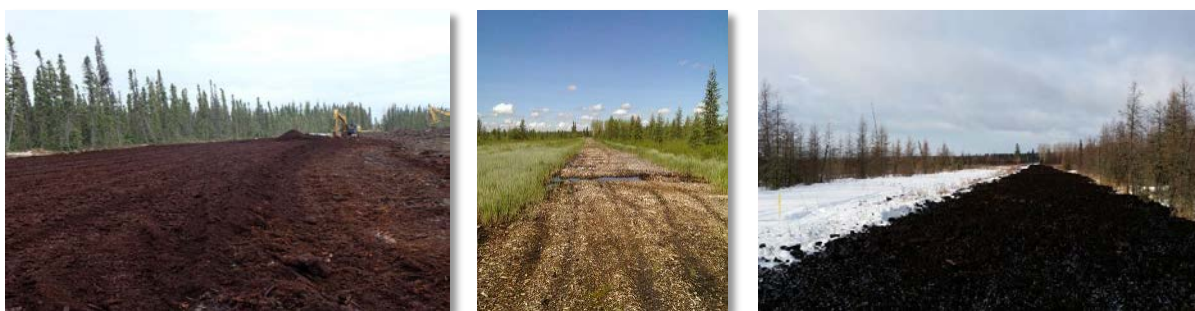
Figure 6. (Left) Inversion trial #2 as the pad is being removed and peat being inverted. (Middle) the chip winter road before reclamation; (Right) The chip winter road after the peat inversion.
