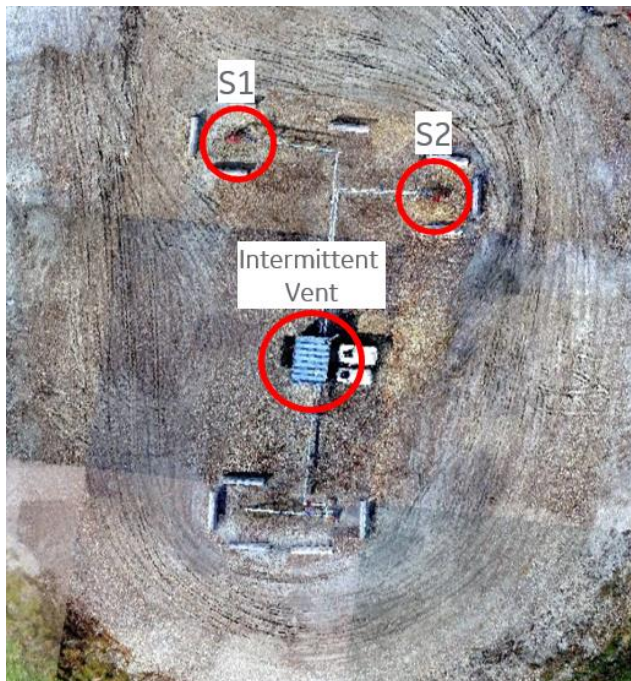
Figure 14. Leak Source Locations at Wellsite
