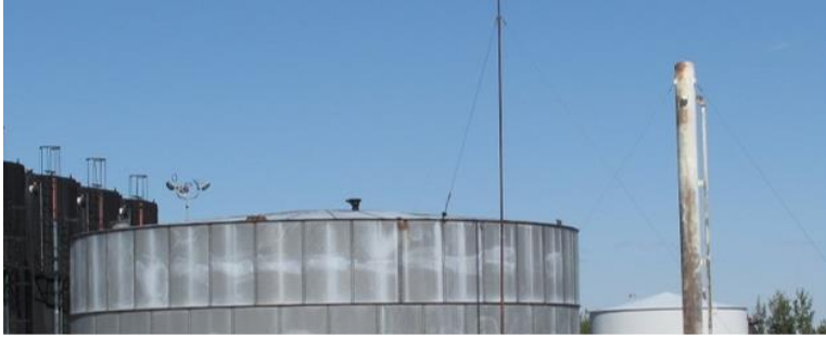
LSD 8-2 Storage Tanks Camera Image
