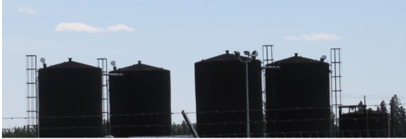
LSD 12-31 Storage Tanks Camera Image
