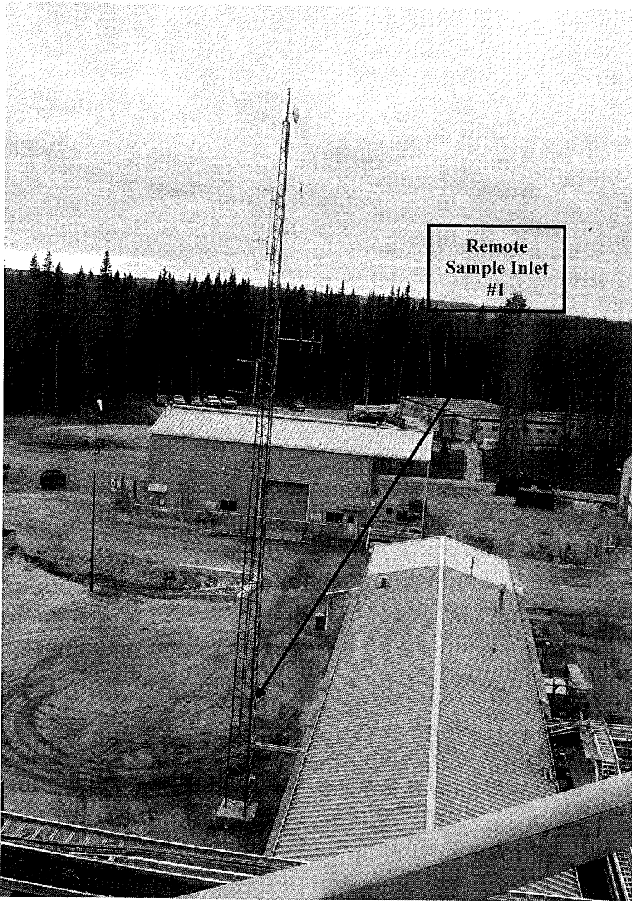
Figure 2: A picture of the remote sampling inlet #1 on the radio tower by the control room.
