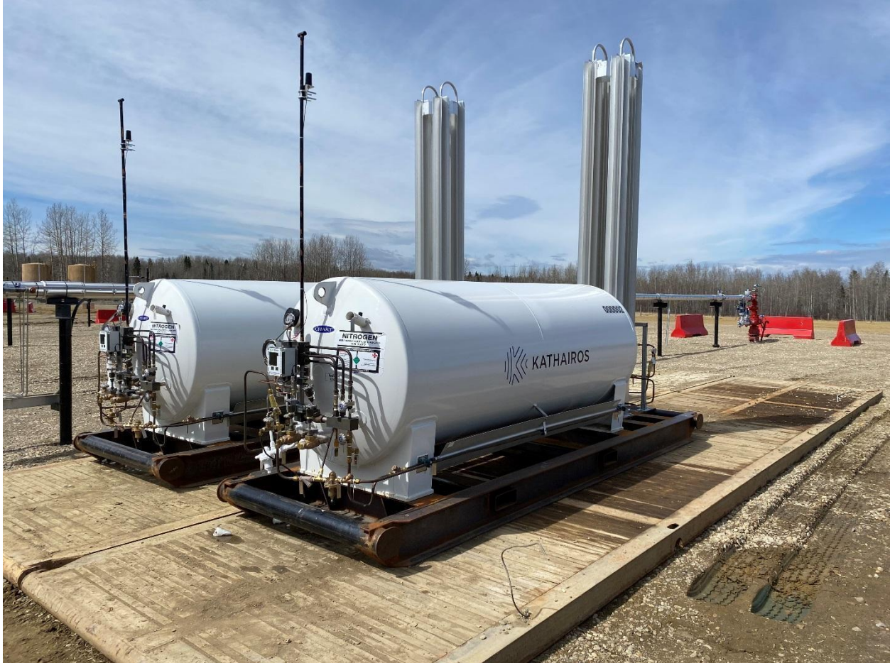
FIGURE 3: TWO HAND-BUILT NITROGEN DEMONSTRATION UNITS
