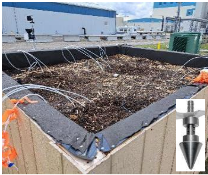
AMS soil gas probe tips were installed at 21 locations within cell
