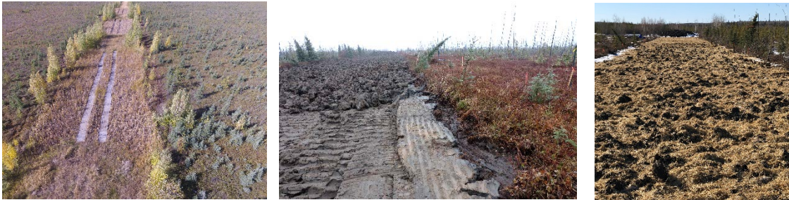
Figure 17. Partial Mineral Fill Removal – JACOS Road
