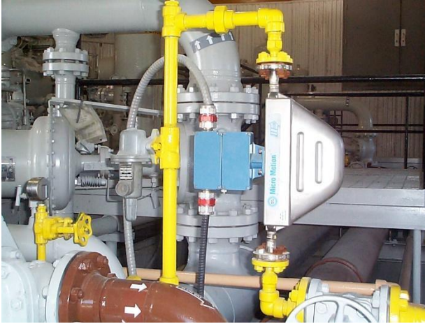
Micromotion ® Coriolis mass flow meter
