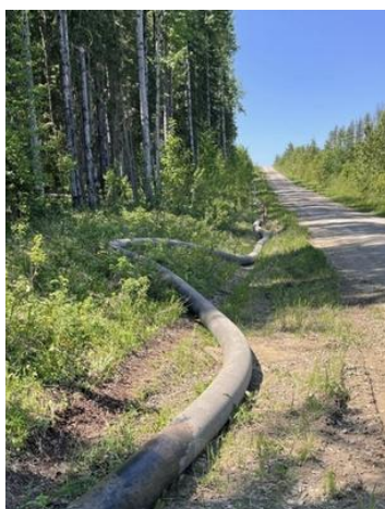
Temporary surface pipeline field verification
